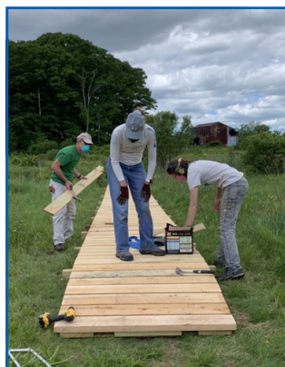
Swallows Field Boardwalk Build at PHP.
