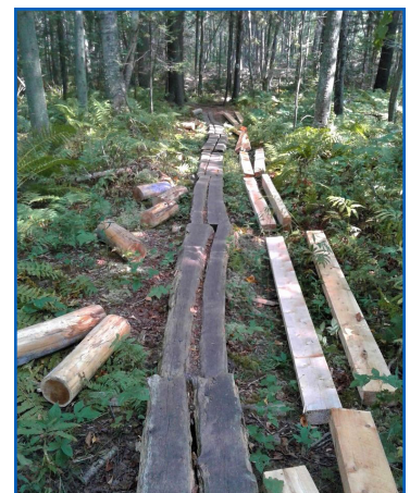
Replacing Bog Bridges at LRF.
