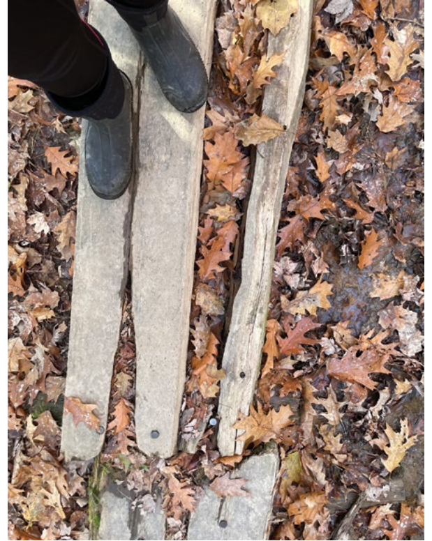
Rotted bog bridges on the Bird Trail.
